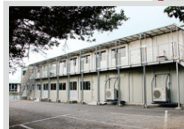
市役所の一部が仮設庁舎へ移転 The city office moved to a temporary building
